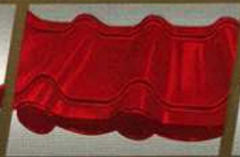
Edge Cap as Installed
